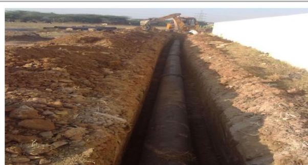
Providing Comprehensive Underground SEWERAGE Scheme and Supplying ,Laying and Testing 350 Dia at Thirumazhisai to CMWSSB, Chennai
